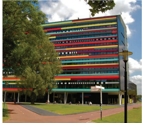
28. Utrecht University campus developed to accommodate the growth of one of the Netherlands' leading Universities
