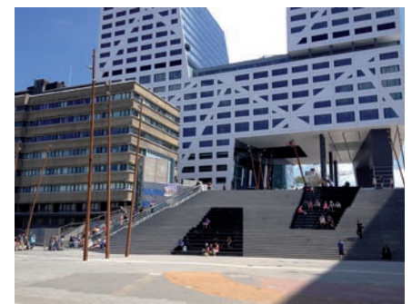
92. Realised new station entrance with new Townhall as new programme and bike storage underneath station entrance
