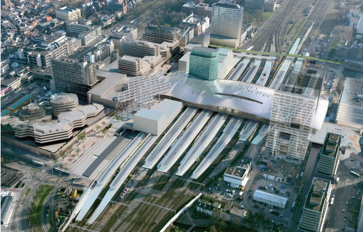
93. New Station (under construction) linking both sides of the city centre and including HST connection on 'classic' rail (and HSR reservation)
